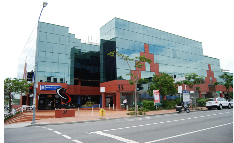
APNIC's Milton office
